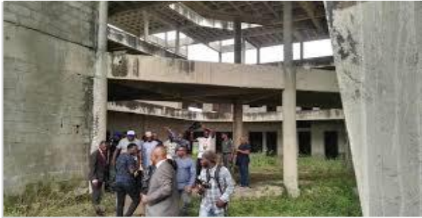
Completion of Civic Centre in Ado Ekiti (N700 Million)
