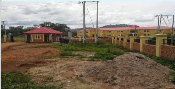
Construction Completion of Oba Adejuyigbe Hospital in Ado Ekiti (N2 Billion)
