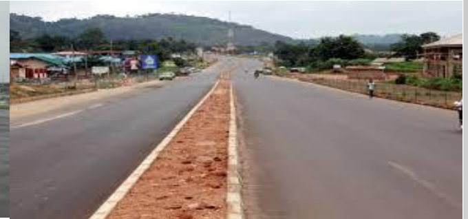
Construction of New Iyin Road in Ado –Iyin Ekiti (N4 Billion)
