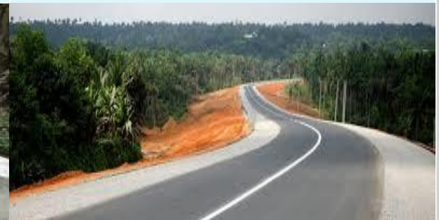
Rehabilitation of Ado-Afao Ekiti Road (N730 Million)
