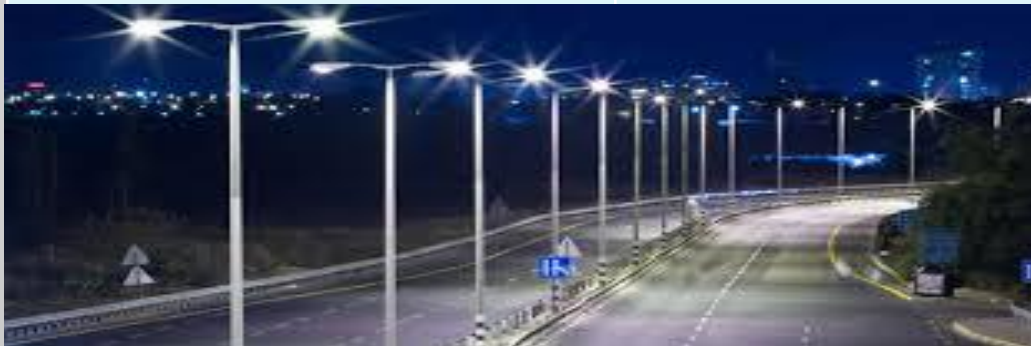
Dualization of Ikere Township Road Phase III (N200 Million)
