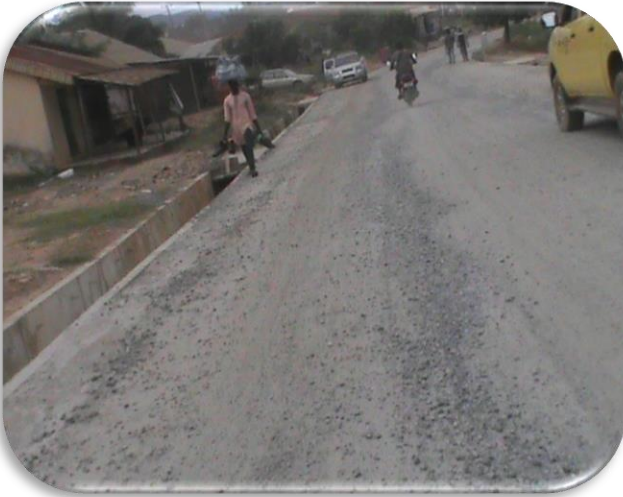
Part of Deeperlife-Ajebamidele roads construction covered with stone base
