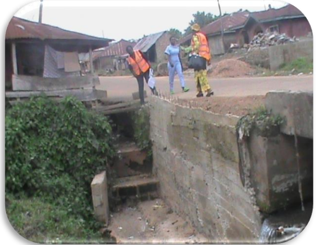
Construction & backfilling of road drainage/cross culvert
