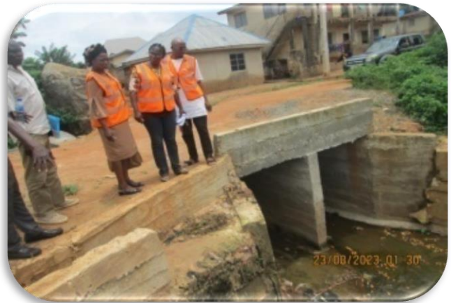
Construction of double cell culvert
