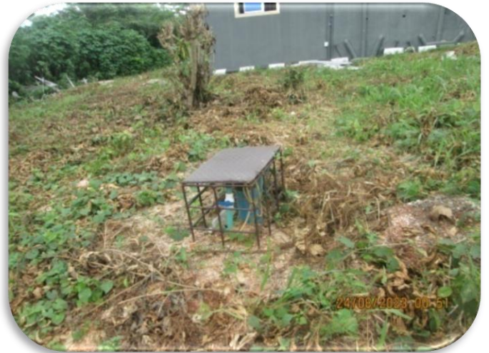
Drilling of borehole with installation of 2 HP Substantive pump with casing
