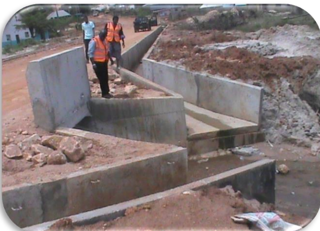
Construction of line drainage & cross Culvert along Deeperlife-Shepherd
