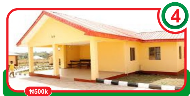
Construction of Primary Health Centres in the State
