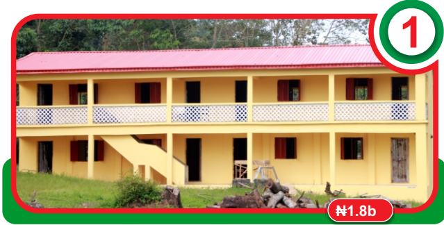
Construction of classrooms for Primary and Junior Secondary Schools across the State
