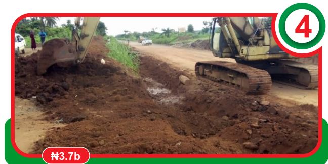
Rehabilitation of 36.8km Itawure-Okemesi-Ijero Road
