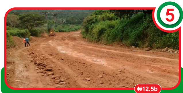
Construction of Rural/Farm Access Roads across the State
