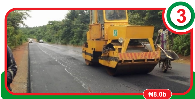
Re-construction of 15km Awo-Ara-Ijero Road
