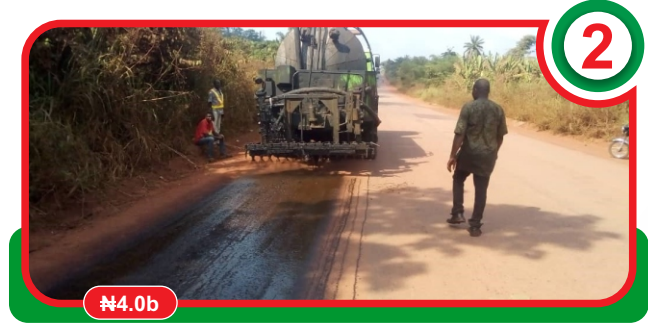
Construction of Oke Ayedun-Ipao-Oke Ako-Irele Road
