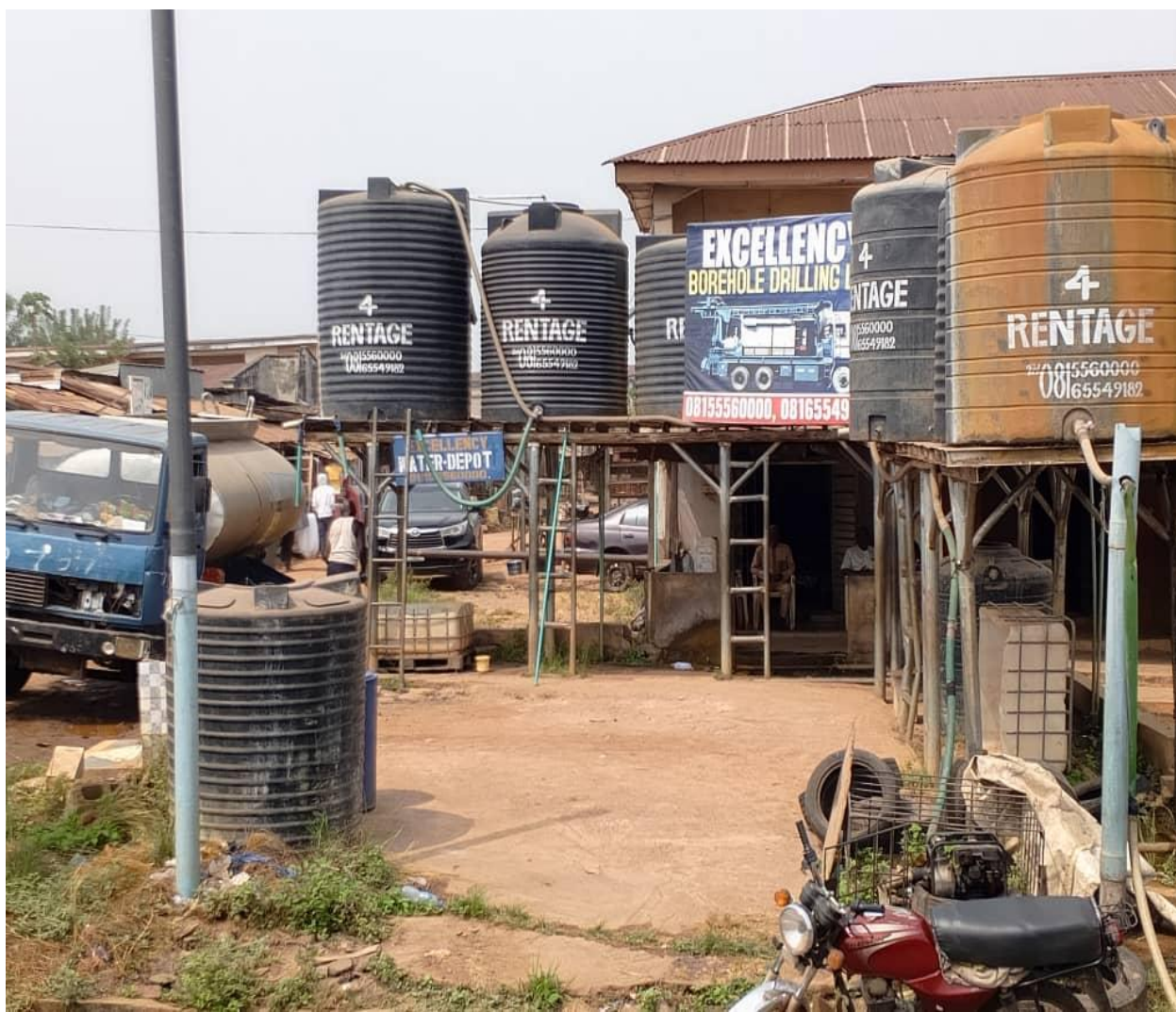
Figure 14: Private borehole small water supply scheme in Ado Ekiti
