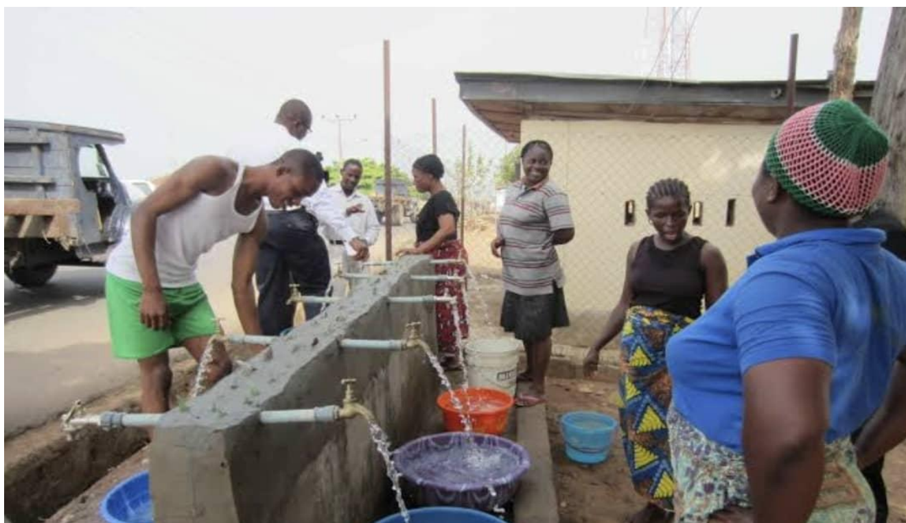
Figure 4: Public Water Supply Standpoint in a Ekiti State Small Town community
