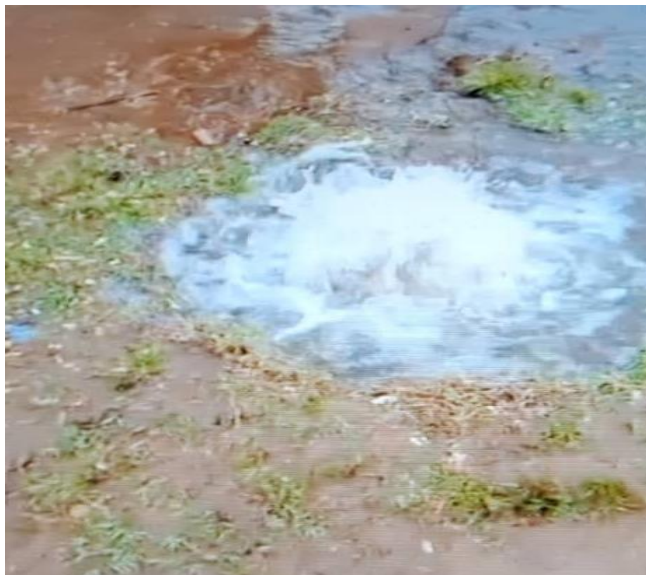
Figure 1: Urban Water Supply (EKWSC) Transmission and Distribution Pipeline burst (NRW)
