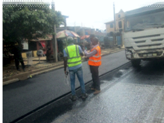
Inspection of Ado Township Road Rehabilitation
