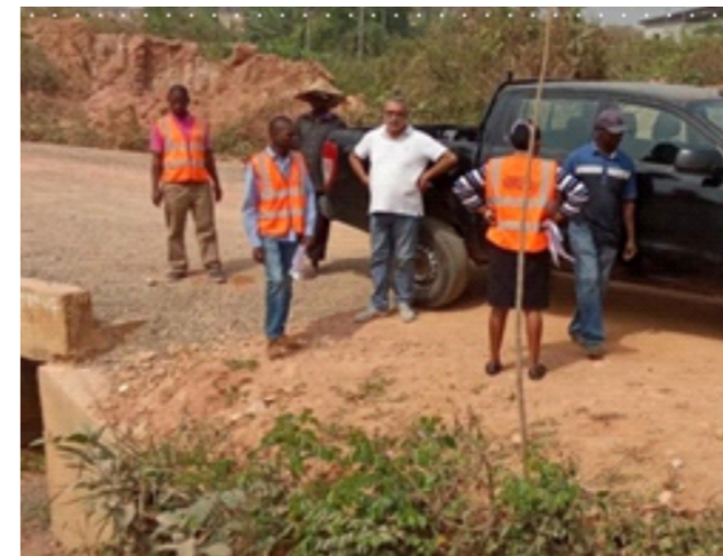
Inspection of GRA Phase-3 Road construction
